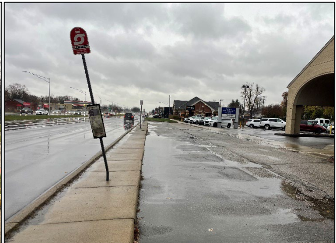
Stop at Woodward Avenue and Vinton Road in Berkley placed in the middle of the sidewalk.
