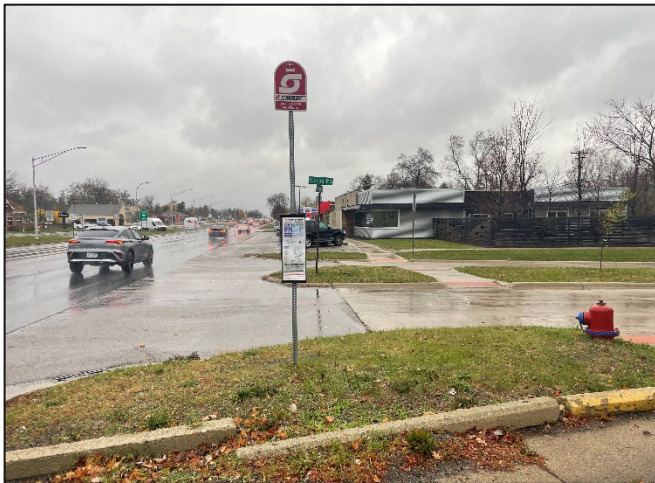
Stop at Woodward Avenue and Edgewood Boulevard in Berkley placed in road verge on uneven surface.
