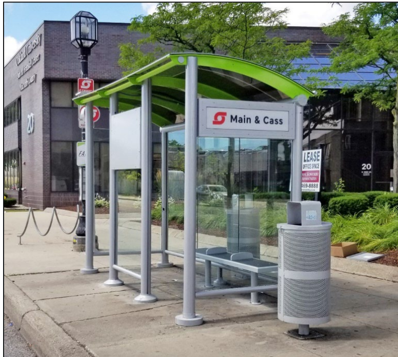
Shelter at South Main Street & Cass Avenue in Mt. Clemens, MI
